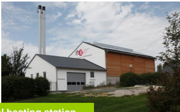
Central heating station
